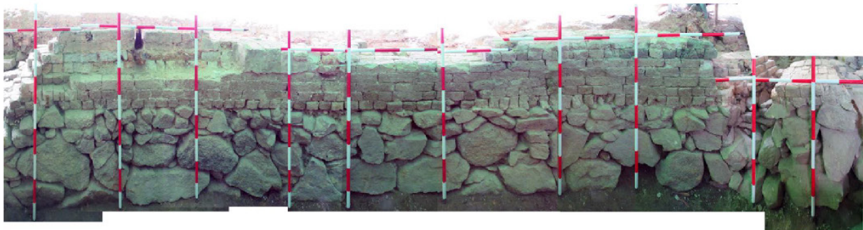
Figure 17 View of Area NE village wall (looking south), note the many smaller stones on top of the stone village wall and row of flat and upright stretchers on top of the leveller to create base for brick wall.
