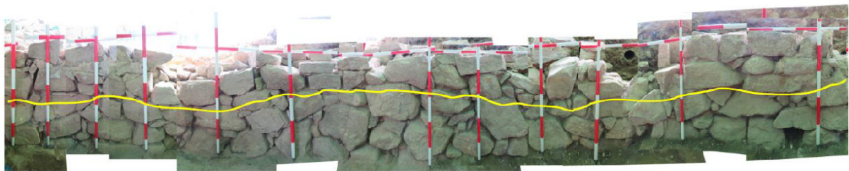
Figure 8 Yellow line shows the approximate division between older and newer stone village wall construction in Area NC; looking south.
