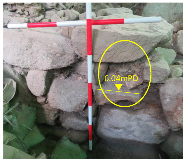
Figure 33 Drain outlet at Lane 6
