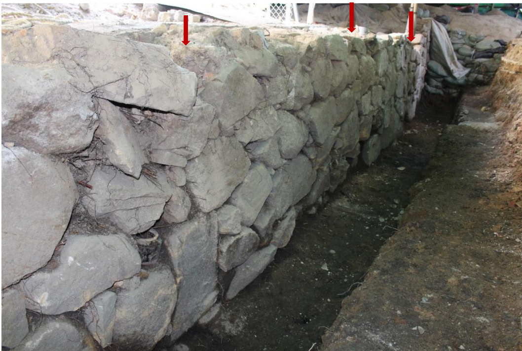
Figure 40 South village wall showing possible sections in construction.
