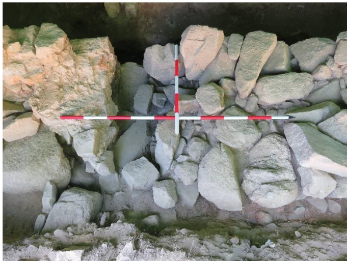
Figure 26 View of disturbed old stone drain; looking south.
